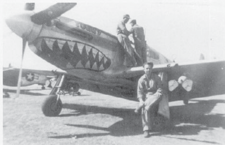
Tommy , a P-51C that was assigned to the Chinese-American Composite Wing, carries dual cluster bomb units under the wings. The CACW was based at Pelshyl, China during 1944. (James V. Crow)
