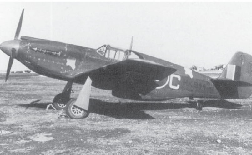
At least one additional A-36A found its way into the RAF. HK 944 was assigned to the Communications Squadron at Foggia during November of 1943. The "patches" on the fuselage are gas detector panels. (Howard Levy via R.L. Ward)
