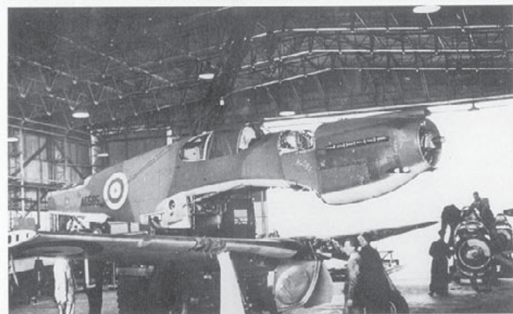
All the Mustang Is were built at North American's Inglewood plant, test flown, then disassembled, crated up, and sent to England by ship. This Mustang I was being reassembled at RAF Burtonwood. (NAA)
